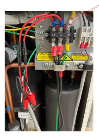
4. Using wire nuts, attach power wire to indoor units to inline fuses. Connect ground wire to to indoor units to ground connection on outdoor unit as shown.
