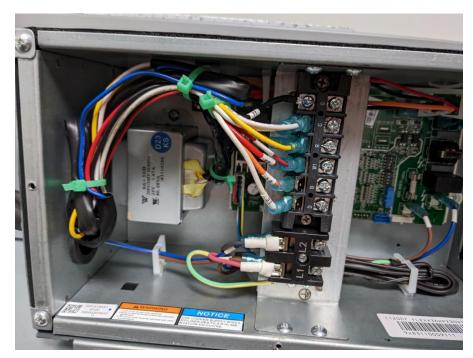
Disconnect line voltage from L1 and L2 permanently before installing an electric heat kit to prevent a high voltage short.
