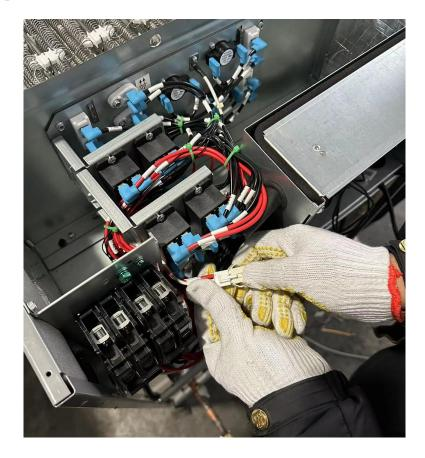
6. Connect the terminal of the electric heater.
