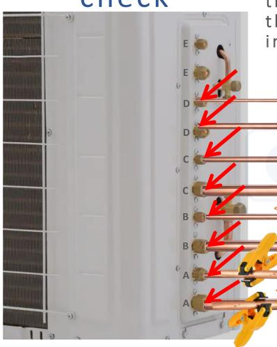
With system operating in cool mode take temperature reading at the large and small lines at the indoor and outdoor units. You should have less than 4°difference between indoor and outdoor on the same line. If more than 4° there is a restriction in the circuit
