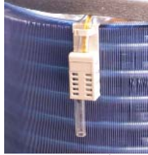
Outdoor Sensor, (mounted on outside of coil)
